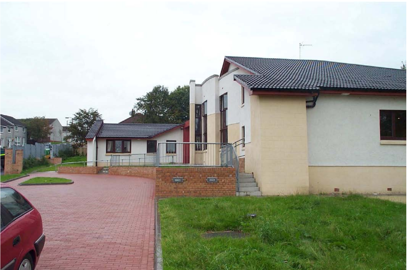
Car parking and garden access
